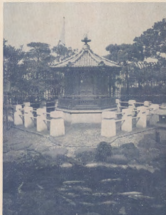
SHRINE ON ROOF OF TAKASHIMAYA DEPARTMENT STORE
